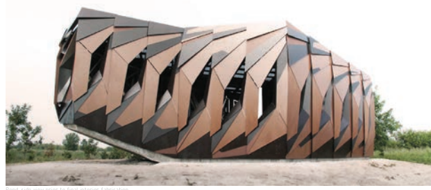
Flood-side view prior to final interior fabrication
